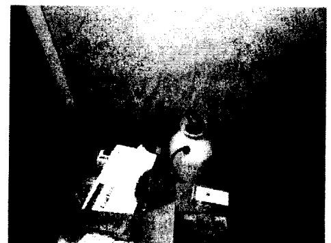
Mold on wall
